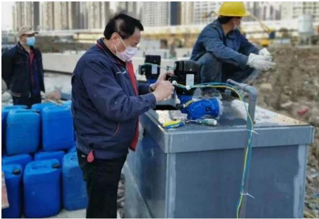
Figure 3 Renovation for sewage treatment at a Fangcang shelter Hospital ( http://www.sasac.gov.cn/n2588025/n2641611/n4518442/c13881088/content.html )
