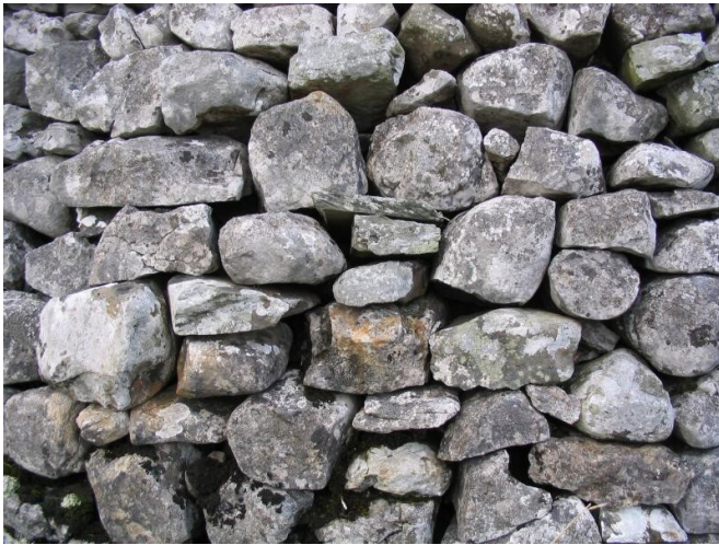
Figure 1 Dry stone wall. Credit: Lupin at English Wikipedia (CC BY-SA). http://upload.wikimedia.org/wikipedia/commons/1/10/Dry_stone_wall_in_the_yorkshire_dailes_detail.jpg
